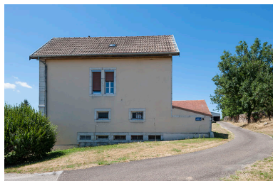
Façade est. Phot. Jérôme Mongreville IVR43_20152501631NUC4A
