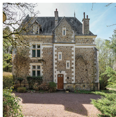
Façade nord-est. Phot. Pierre-Marie Barbe-Richaud IVR26_20195800047NUC4AQ
