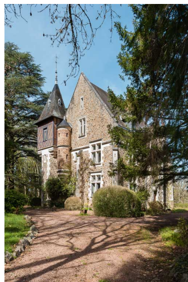
Façade sud-est. Phot. Pierre-Marie Barbe-Richaud IVR26_20195800036NUC4A
