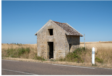
La cabane de trois quarts. Phot. Nicolas Waltefaugle IVR26_20268900267NUC4A
