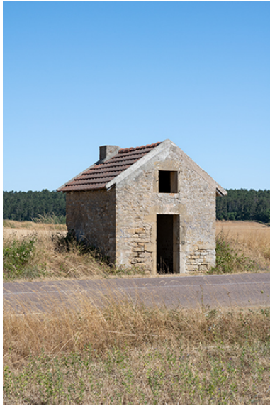
La cabane de trois quarts. Phot. Nicolas Waltefaugle IVR26_20268900271NUC4A
