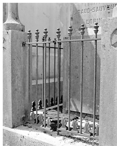
Grille. Phot. Yves Sancey IVR43_20033901137X
