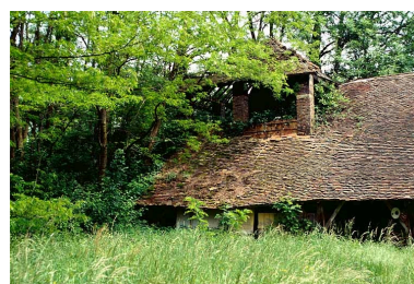
Four industriel. Phot. Jérôme Mongreville IVR43_19963900503ZA
