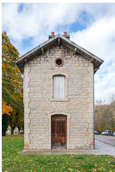
Mur-pignon sud. Phot. Nicolas Waltefaugle IVR43_20253900351NUC4A
