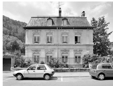
Elévation antérieure. Phot. Yves Sancey IVR43_20033900114X
