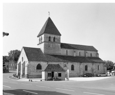
Elévation gauche. Phot. Michel Rosso IVR26_20037101549X
