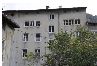
Elévation postérieure. Phot. Yves Sancey IVR43_20093900125NUC2A
