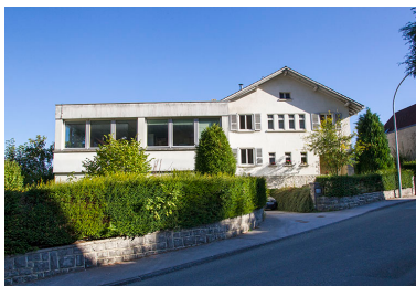
Façade antérieure. Phot. Yves Sancey IVR43_20132502353NUC2A
