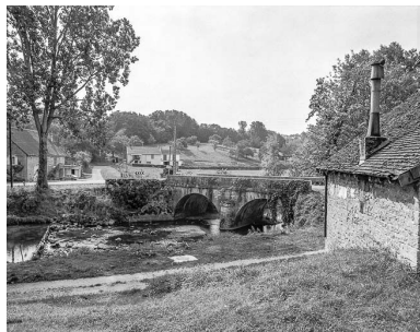
Face amont. Phot. Yves Sancey IVR43_19843900109X
