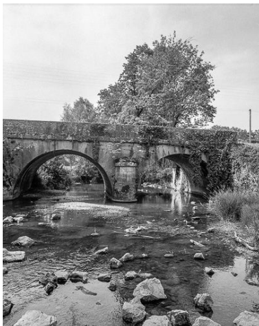
Face amont. Phot. Yves Sancey IVR43_19843900110X
