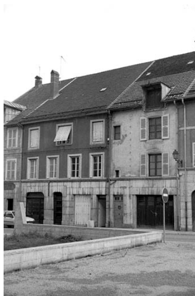
Logement patronal. Phot. Laurent Poupard IVR43_19913901307Z
