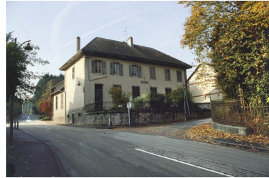
Façade nord. Phot. Yves Sancey IVR43_20009000782ZA
