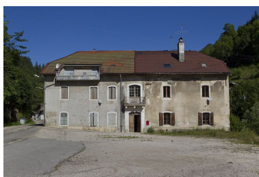
Logement patronal. Phot. Yves Sancey IVR43_20103900663NUC2A
