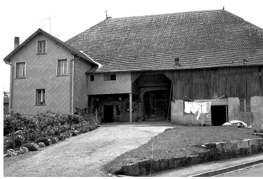
Façade postérieure. Phot. Gilbert Poinot IVR43_19752500874Z
