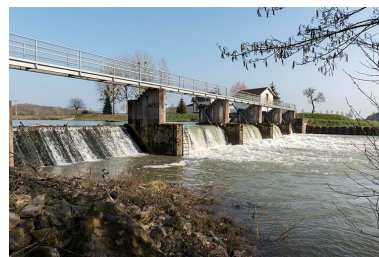
Le barrage mobile de Montureux-lès-Baulay. Phot. Sonia Dourlot IVR43_20167000288NUC4A
