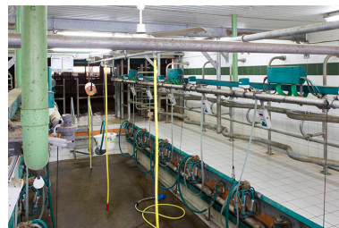
Salle de traite. Phot. Sonia Dourlot IVR43_20143900894NUC2A
