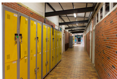
Circulation intérieure. Phot. Sonia Dourlot IVR43_20143900808NUC2A
