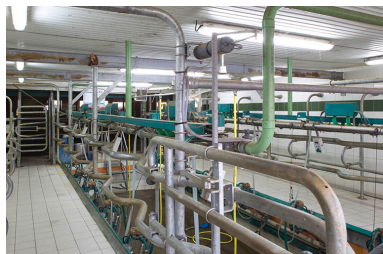
Salle de traite. Phot. Sonia Dourlot IVR43_20143900895NUC2A
