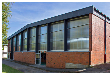
Façade nord du gymnase. Phot. Sonia Dourlot IVR43_20143900840NUC2A
