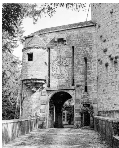
Pont-levis. Phot. Dominique Dominguez IVR43_19807000280X
