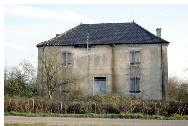
Logement patronal. Phot. Laurent Poupard IVR43_19883900709ZA
