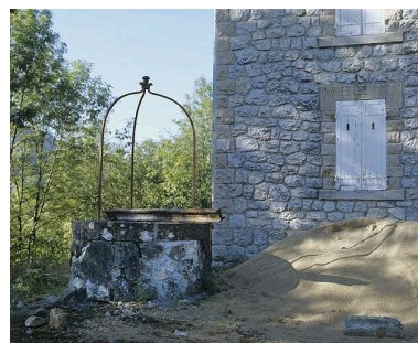
Puits. Phot. Yves Sancey IVR43_20043900345XA
