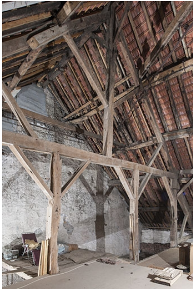
Charpente. Phot. Jérôme Mongreville IVR43_20127000447NUC4A
