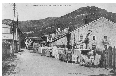
Molinges - Usines de Marbreries. Phot. Yves Sancey IVR43_19973900032X
