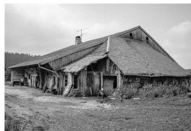
Façade postérieure. Phot. Gilbert Poinot
