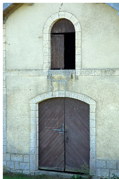
Portes du magasin. Phot. Sonia Dourlot IVR43_20157001518NUC2A
