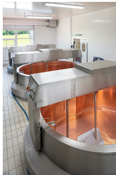
Les trois cuves. Phot. Sonia Dourlot IVR43_20192500949NUC4A
