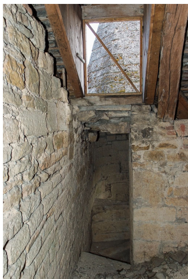
Combles. Phot. Pierre-Marie Barbe-Richaud IVR26_20152100460NUC2A
