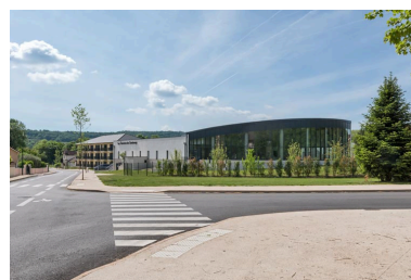
Centre thermal de 2021. Phot. Pierre-Marie Barbe-Richaud IVR26_20222100212NUC4A
