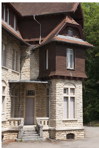
Façade sud. Avant-corps. Phot. Jérôme Mongreville IVR43_20112501321NUC4A
