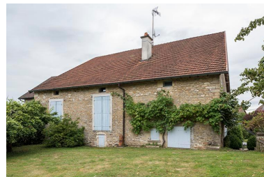
Façade arrière Phot. Sonia Dourlot IVR43_20167001112NUC4A
