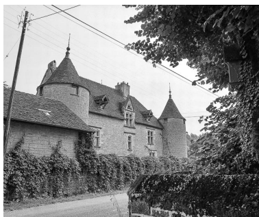
Façade sud Phot. Yves Sancey IVR43_19753901074X
