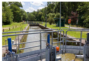
Ecluse n°40, Selles (70). Phot. Sonia Dourlot IVR43_20157000917NUC2A
