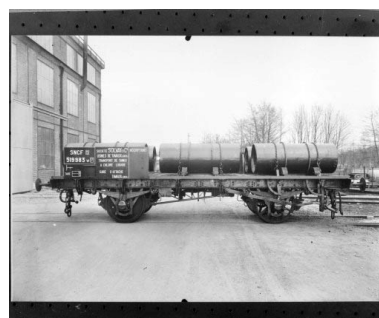
Wagon-citerne servant au transport de chlore liquide. Phot. Jérôme Mongreville, Phot. Charnotet IVR43_19903900082X
