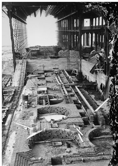
Atelier de caustification : construction des pots. Phot. Jérôme Mongreville, Phot. Charnotet IVR43_19903900059X
