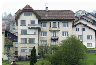
Façade postérieure. Phot. Sonia Dourlot IVR43_20162500904NUC4A
