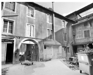
Bâtiment est. Phot. Yves Sancey IVR43_20033900711X
