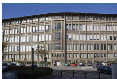
Aile sud. Phot. Yves Sancey IVR43_20092501489NUC2A
