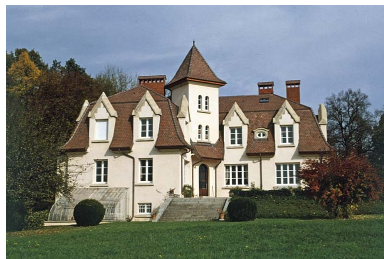
Façades ouest. Phot. Yves Sancey IVR43_20009000853ZA
