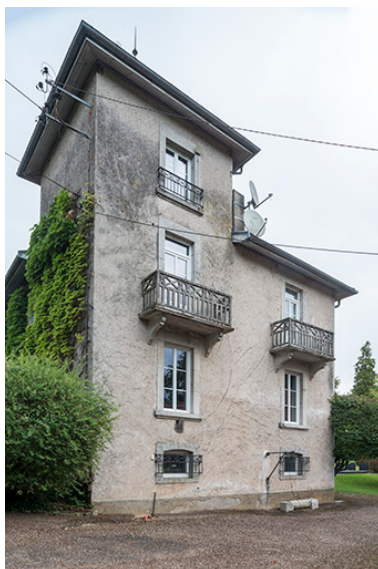
Mur pignon sud. Phot. Jérôme Mongreville IVR43_20177001108NUC4A
