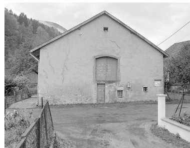
Face nord. Phot. Jérôme Mongreville IVR43_19963901640X
