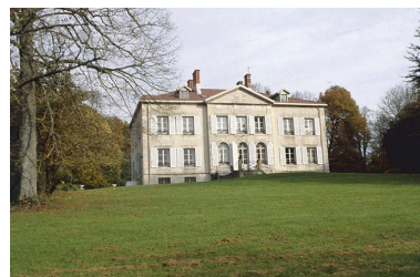
Façade ouest. Phot. Yves Sancey IVR43_20009000869ZA
