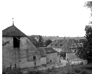
Façade principale. Phot. Yves Sancey IVR43_19843900369X
