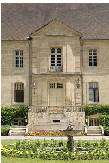
Logis abbatial. Avant-corps central. Phot. Jérôme Mongreville IVR43_20097000681NUC2A
