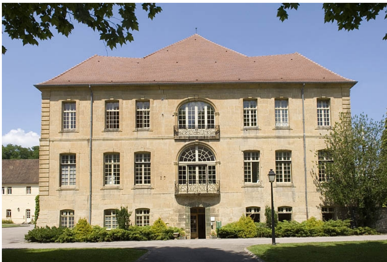
Logis abbatial. Façade sud.
