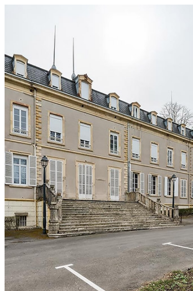
Aile nord, façade. Phot. Pierre-Marie Barbe-Richaud IVR26_20227100027NUC4A
