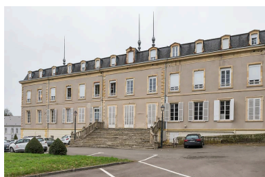
Aile nord, façade. Phot. Pierre-Marie Barbe-Richaud IVR26_20227100049NUC4A
