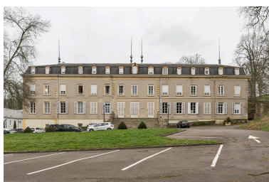
Aile nord, façade. Phot. Pierre-Marie Barbe-Richaud IVR26_20227100048NUC4A
