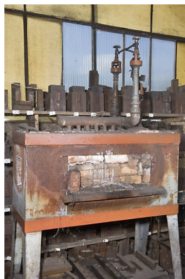
Atelier est. Four à gaz Thermidor. Phot. Jérôme Mongreville IVR43_20087000816NUC2A
