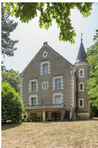
Mur pignon nord-est. Phot. Pierre-Marie Barbe-Richaud IVR26_20195800531NUC4A
