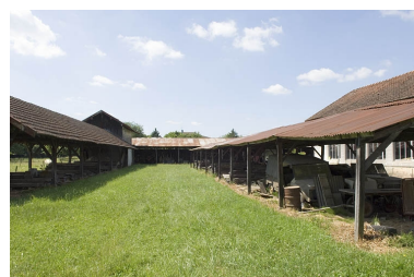
Entrepôts industriels sud. Phot. Jérôme Mongreville IVR43_20097000431NUC2A
