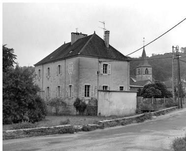
Face postérieure. Phot. Yves Sancey IVR43_19843900223X
