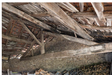
Charpente du cuvage Phot. Pierre-Marie Barbe-Richaud IVR26_20197100257NUC4A
