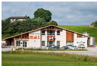
Façade est. Phot. Jérôme Mongreville IVR43_20142501153NUC4A
