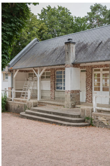
Club-house, entrée. Phot. Pierre-Marie Barbe-Richaud IVR26_20195800419NUC4A
