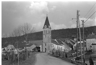
Vue de situation. Phot. Guy Forestier IVR43_19743900506Z
